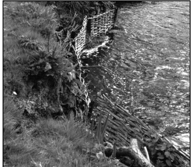
Hazel hurdles can be used to repair the damage done by overgrazing, but erosion will continue if the cause is not dealt with by fencing livestock or reducing stocking densities.
