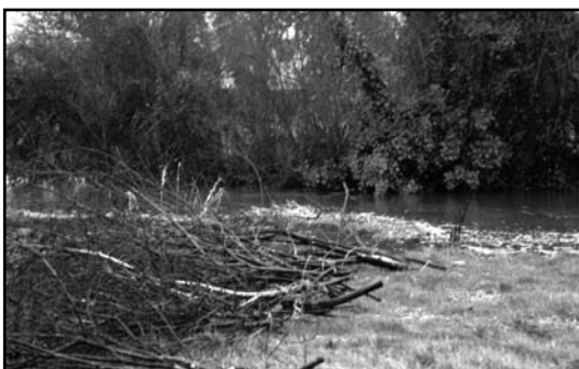
Faggots provide a flexible tool for bank protection.
