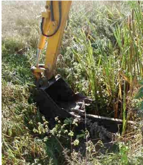
A digger and bucket can be used to lift turfs containing reed roots
