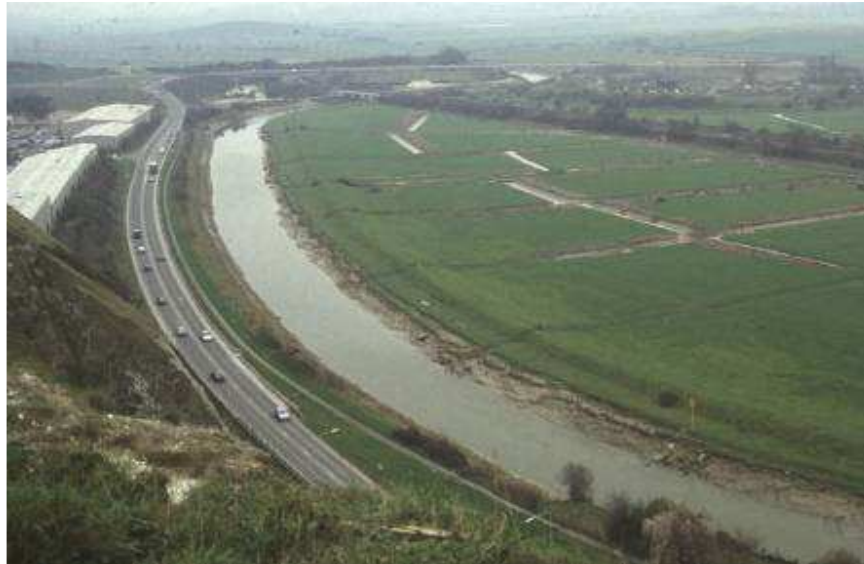
A river which has been straightened and confined between a road and a large embankment. When the river floods, water gets 'stuck' in the river channel and can't go anywhere. It backs upstream and can cause flooding.
