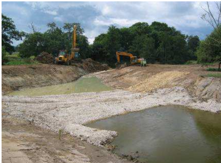
The Environment Agency restoring a river channel which had silted up entirely.
